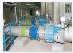
carbon dioxide, active charcoal and sodium sulphite dosing device including pipelines. Also, new parts of the potassium permanganate, limewater and aluminium sulphate pipelines were installed.
