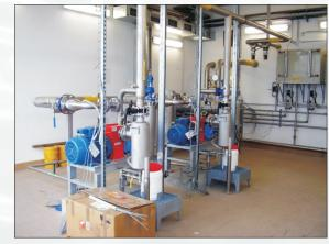
Three boilers including accessories - one for natural gas, one for biogas and one for natural gas or biogas combustion - are installed as a thermal energy source to cover any treatment plant heat losses.
